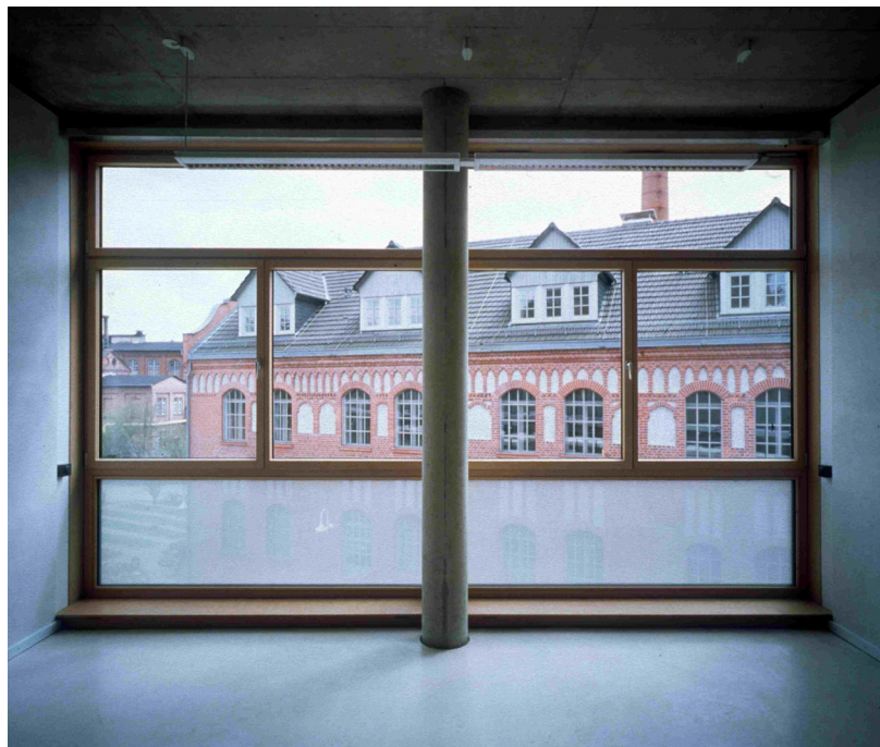
Figure 3 Inside view of an office room (Meyer 2001)
