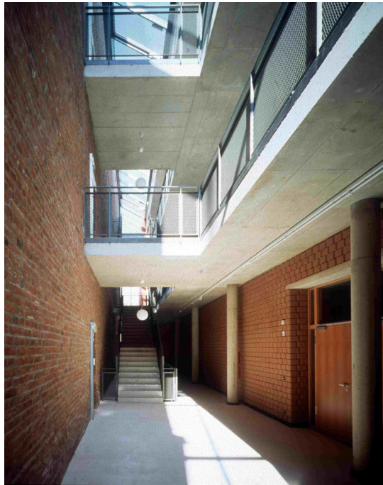
Figure 7 View inside the atrium, it shows the open thermal masses and the internal clay wall used for all the installations (right hand side) (Meyer 2001)
